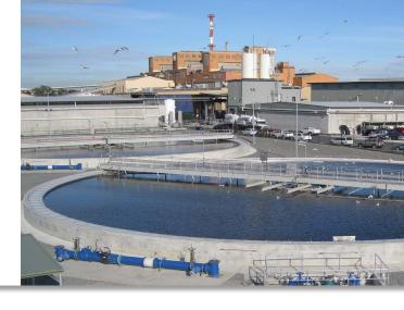
Gibson Island STP was upgraded in 2008 as part of the Western Corridor scheme in Brisbane, to allow for the advanced treatment of secondary effluent to enable reuse.
