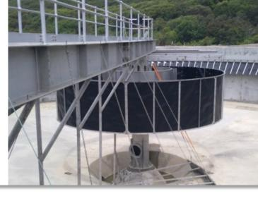
• The scum skimmer is a hinged stainless steel blade with neoprene squeegee, supported from the bridge which skims the water surface adjacent to the scum baffles.
