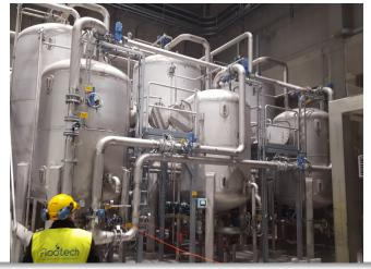
In 2017, Hydroflux completed a major upgrade to a demineralised water treatment plant for one of Australia's largest pulp & paper facilities. The upgrade involved the replacement and redesign of the existing cation and mixed bed ion exchange processes, including the supply of new specially designed SS316L Hydroflux FlooIX exchange vessels. The FlooIX system has a production capacity of 250m<sup>3</sup>/hr of high purity water used for steam generation.
