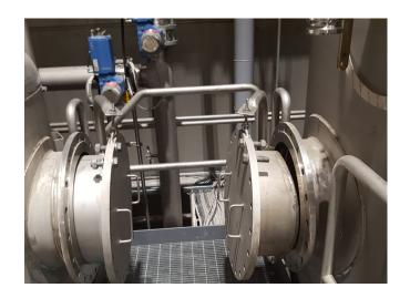
attractive for high flow demineralized water treatment systems. The new facility features Hydroflux FlooIX ion exchange vessel, manufactured entirely from stainless steel. The design includes a customizable set of internal chemical regeneration lateral diffusers to allow the vessel to be used in different services. This was one of the key advantages in the Hydroflux design, as it allowed the client the flexibility to modify the vessels use to suit future process changes.
